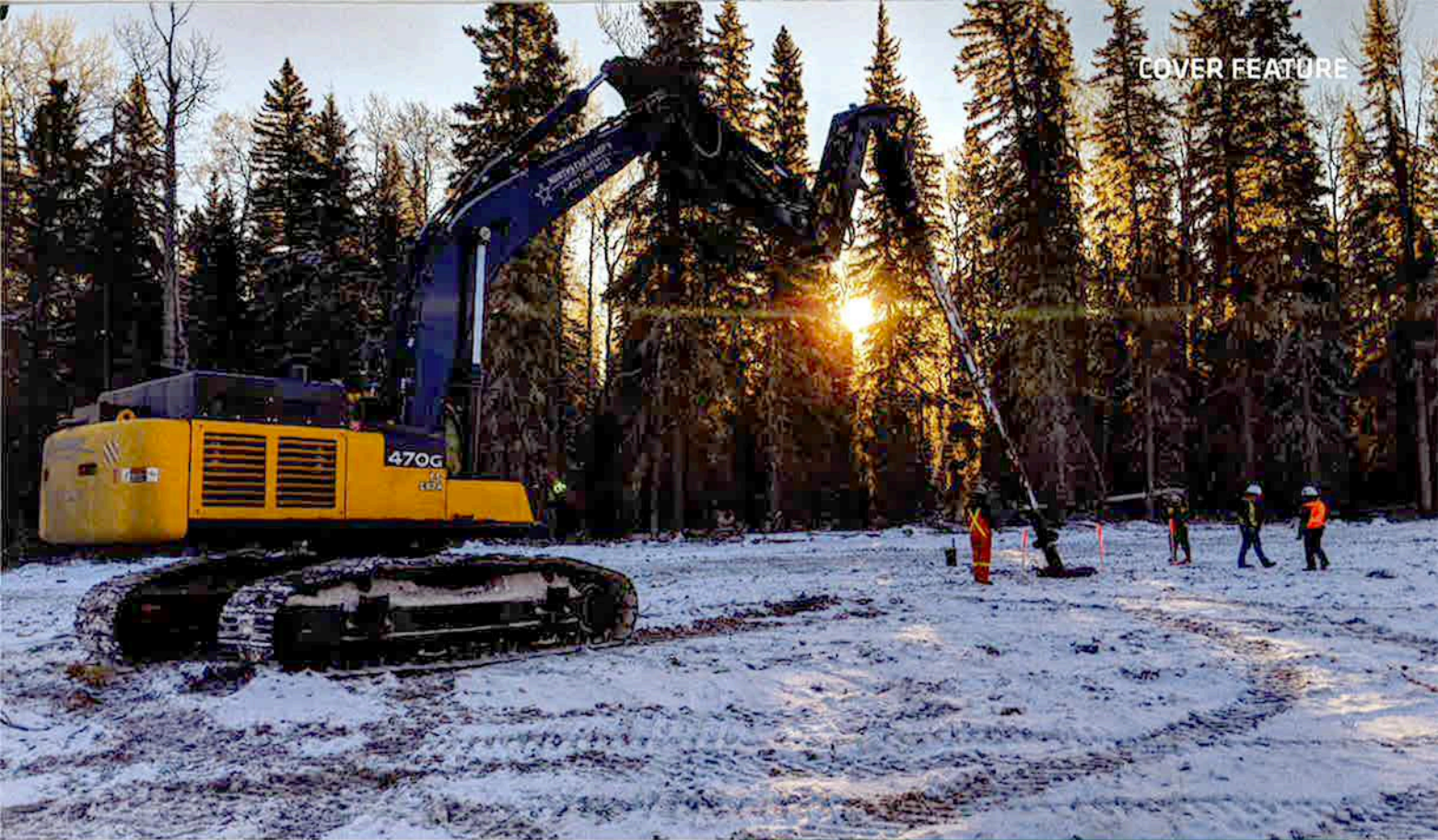
Helical piles being installed by Northstar Sharp's Exca-Driver
